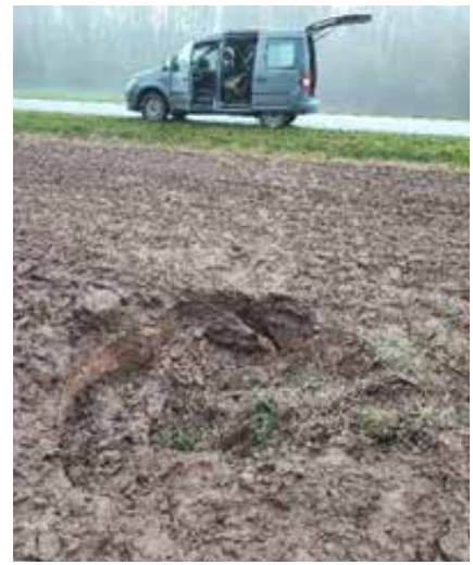
Fig. 6. Forming new sinkhole in Mantagailiškis
