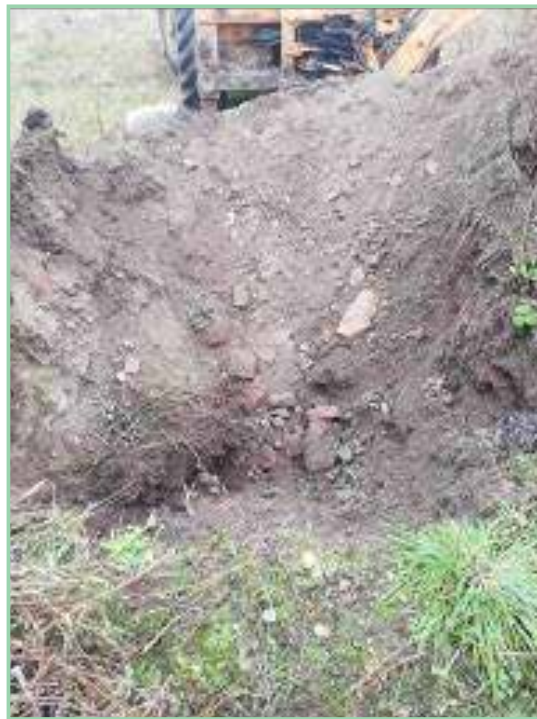
Fig. 6. Construction waste excavated along the profile (Fig. 4).
