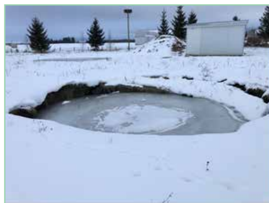
Fig. 8. Sinkhole near the wellfield of Saločiai town (on a orthophotographic map (left) and phenomena causing a risk near the buildings of eldership and gymnasium (photo by A. Lindienė, February 4, 2021).
